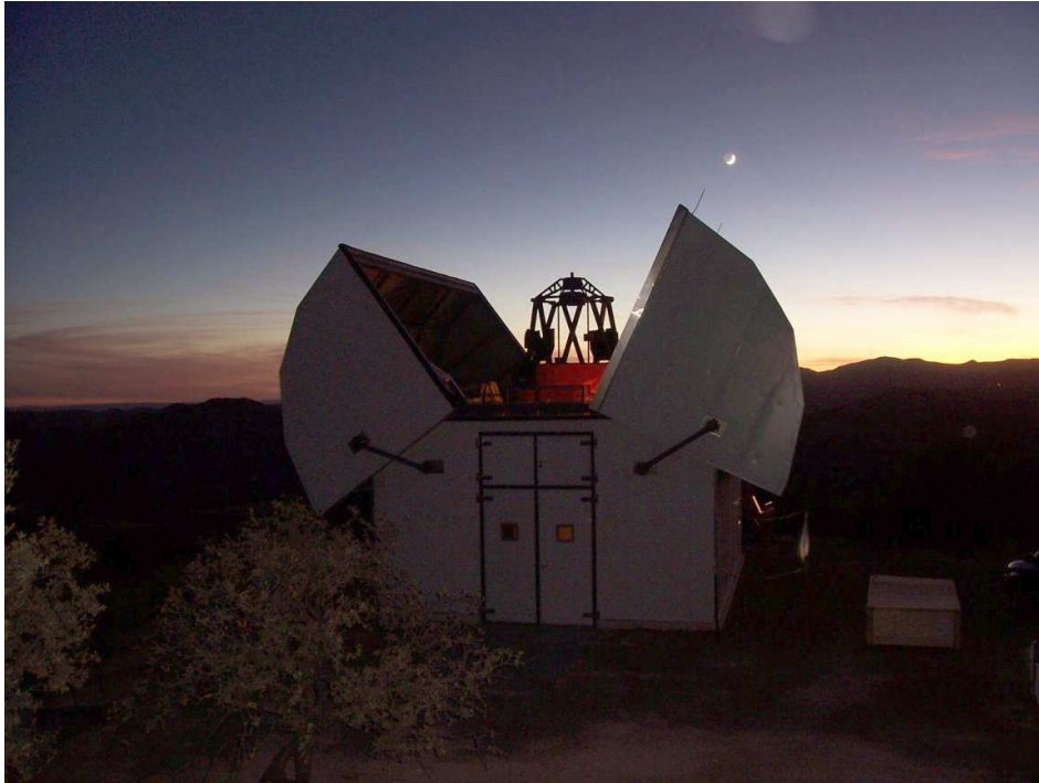
Fig. 2. The partially opened clamshell enclosure reveals the MONET/North telescope at dusk. In this position the enclosure can shield the telescope against wind gusts. In the background the horizon is shaped by lovely Davis mountains of western Texas.
